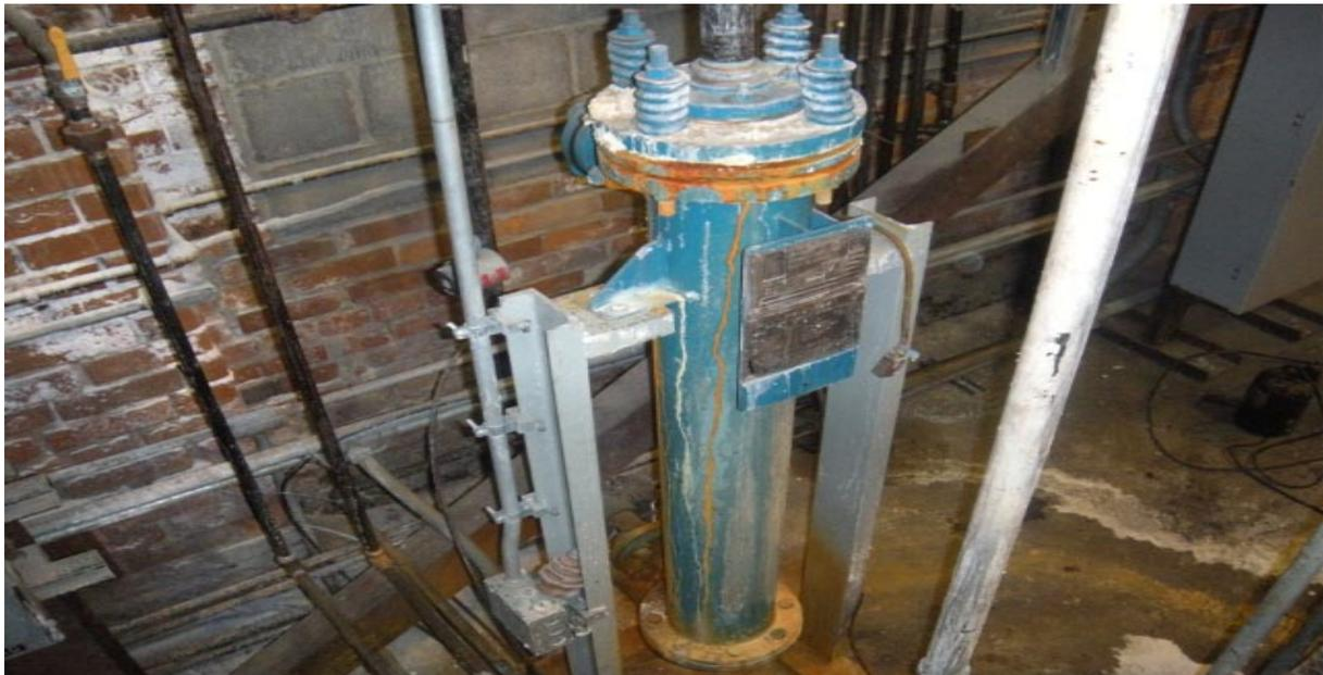
**(10) Heat Exchangers** – Two are utilized, one to heat up the virgin CAC-24 before introduction into the process and the other to keep the process chemistry up to the operating temperature of 135-155°F.
